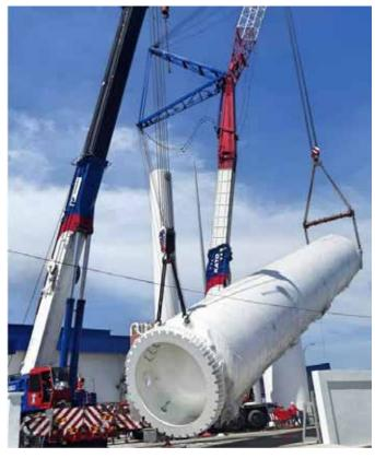
Cryogenic Storage Tank L29.00 m x W4.30 m x H4.45 m 92 ton
