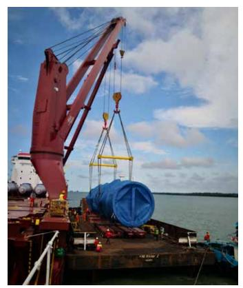
HDS Reactor L38.52 m x W7.20 m x H7.25 m 466 ton
