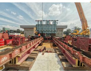
The Transformer was delivered using multi-axle hydraulic trailer from Thailand to the solar project in Perak. Upon arriving at site, we did a jack and skid operation to move the Transformer onto its foundation.
