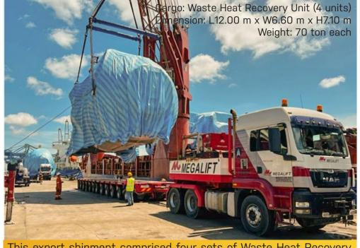
This export shipment comprised four sets of Waste Heat Recovery Units and their accessories of 12 packages each. The cargoes, close to 2,400 FT in total, were transported to Port Klang by our team to catch the conventional vessel to Shandong, China.
