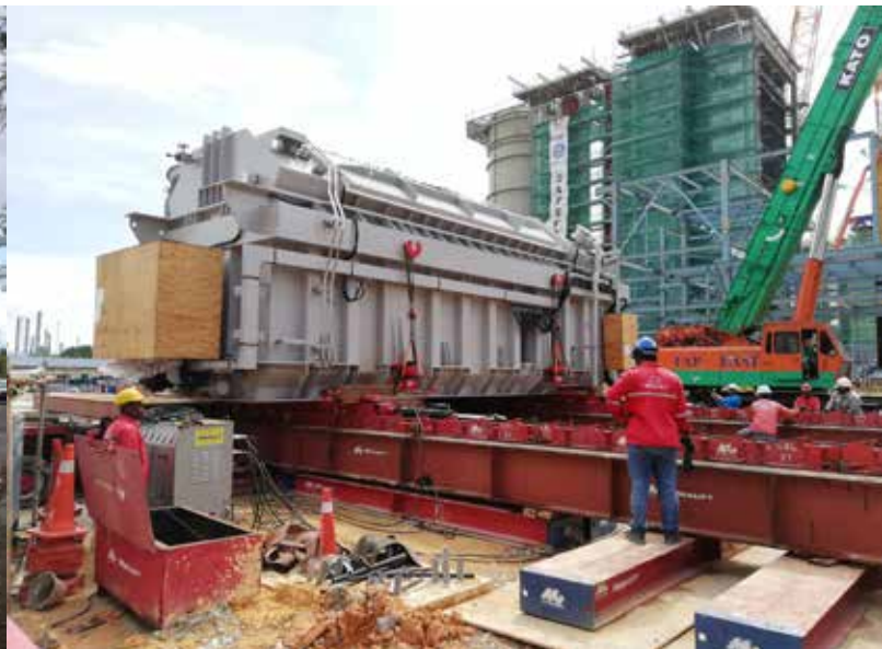
Transportation and jack and skid of Transformer L12.00 m x W4.60 m x H4.52 m | 342 ton
