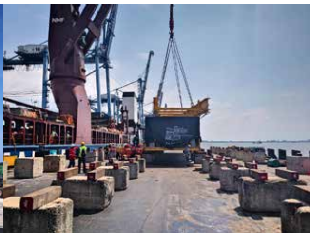
Transportation and jack and skid of Transformer L12.00 m x W4.60 m x H4.52 m | 342 ton
