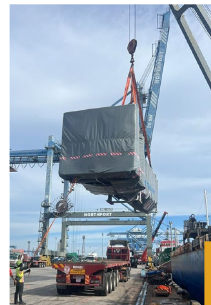
Cargo: Series Tunnel Dimension: 17.65 m x W3.68 m x H3.95 m Weight: 24 ton
