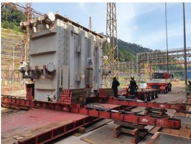
Megalift was tasked to send this unit of Transformer along with its accessories from Manjung to Thailand. At the site, we jacked and skidded the Transformer from its foundation onto our multi-axle trailer. We used our drop deck trailer to cater for its over height. From Manjung, we rode for almost 300 km to Bukit Kayu Hitam before our Thai partner took over.
